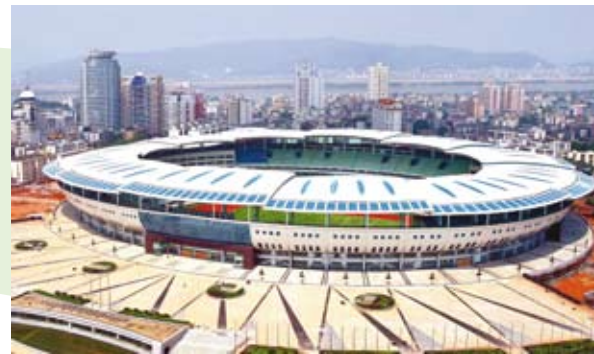
Changsha New Century Sports Centre, Changsha, China
